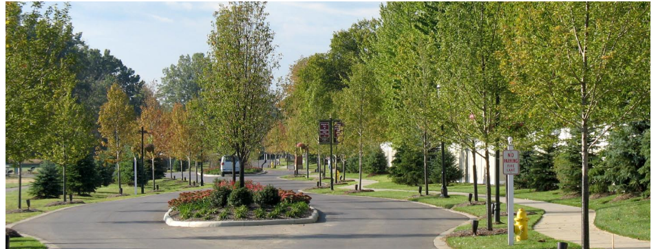
Creative stormwater management helped save on construction costs for the Vintage Club development
