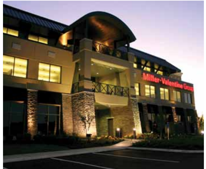
Two Waterstone Place, Offices for Miller-Valentine Group
