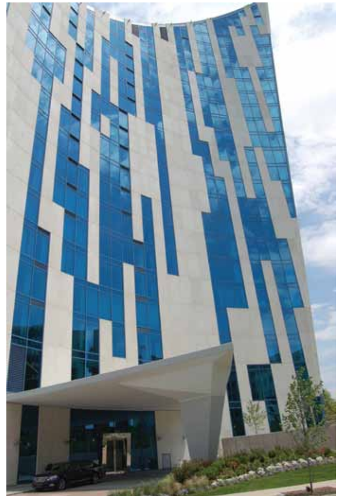
The Ascent at Roebling's Bridge
